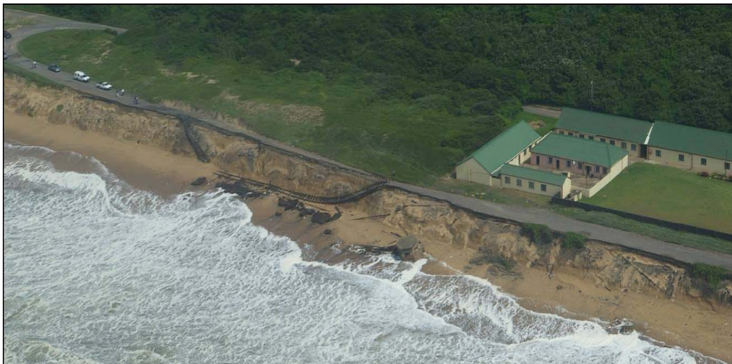
Figure 9: Damage to coastal roads cause by the KZN sea-level rise event of 2007 (Source A. A Mather)
